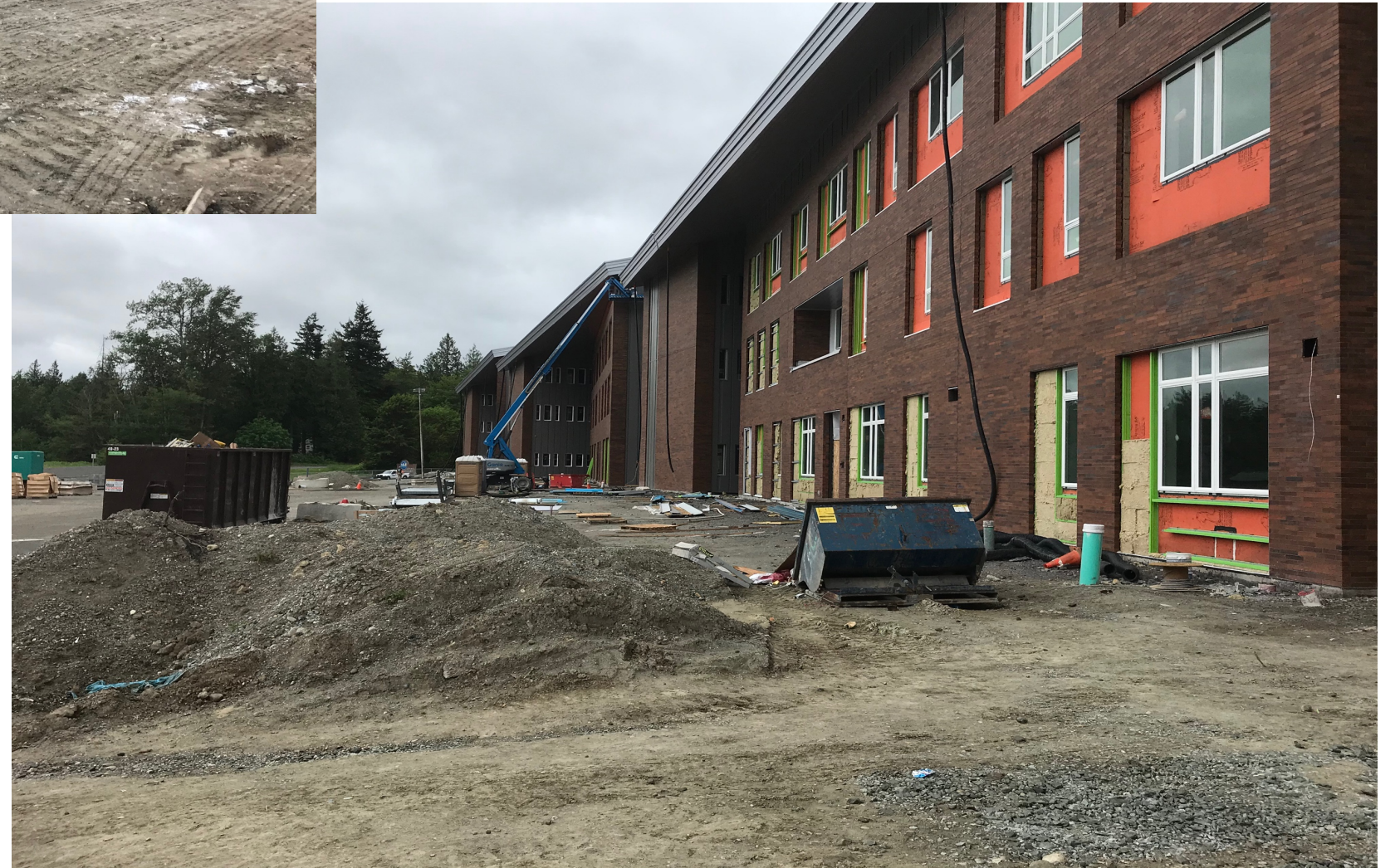
View of south elevation from Commons entry
