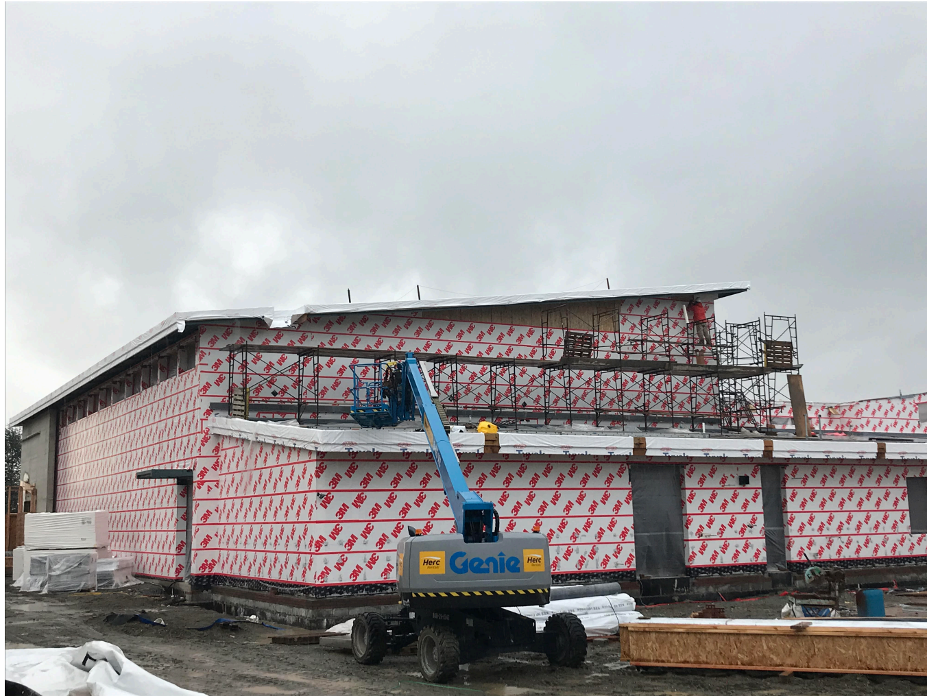
NW View of Gym from Saratoga Classroom
