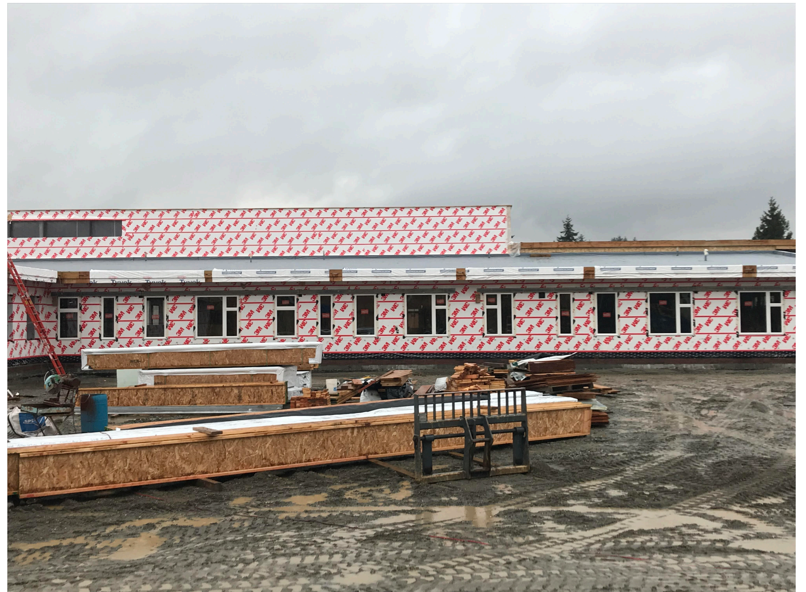
South View of Lincoln Classrooms
