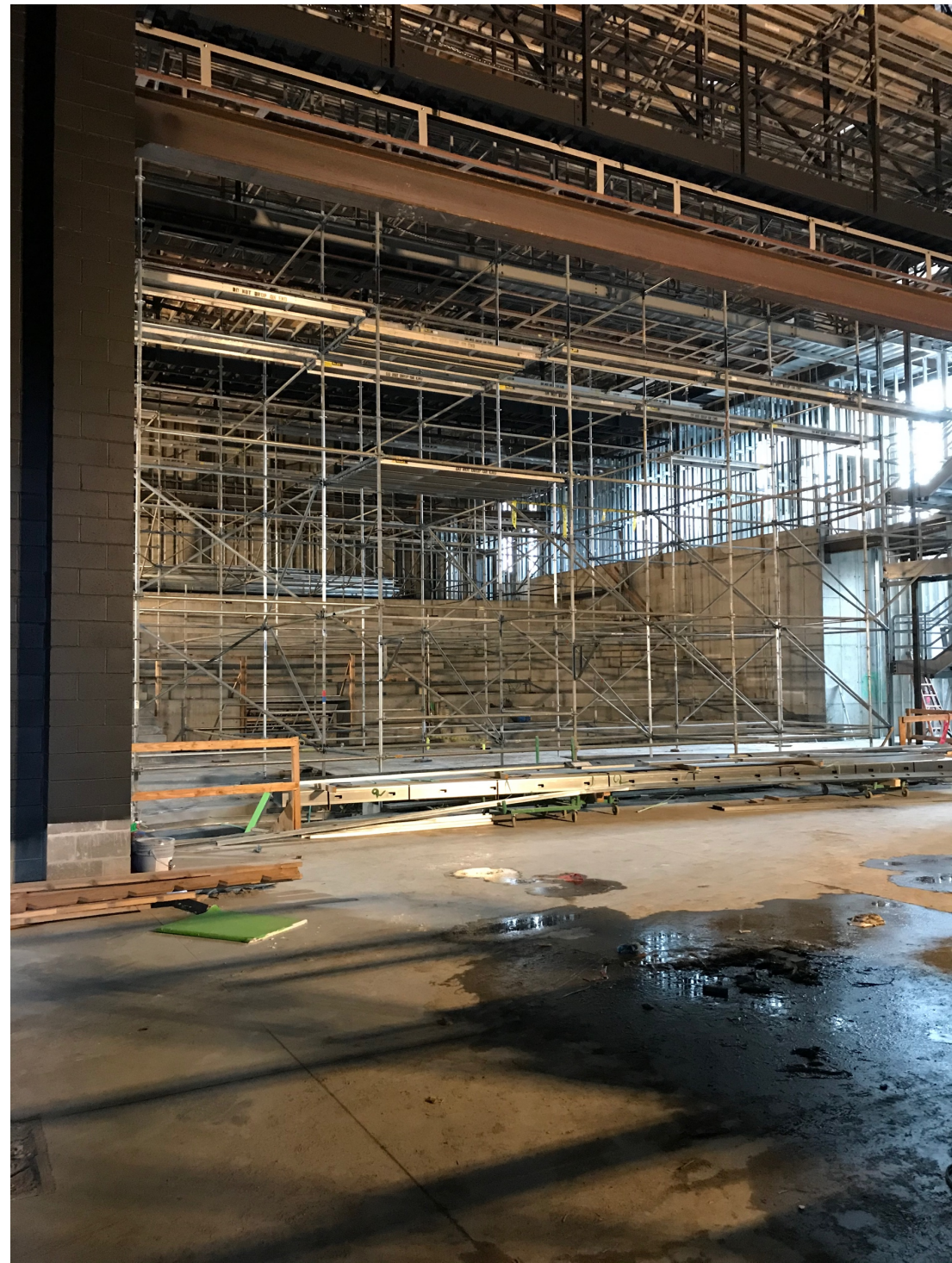
PAC scaffolding from stage
