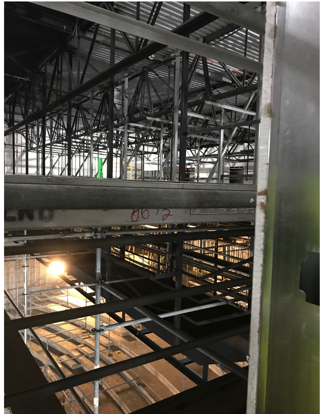
PAC scaffolding from catwalk
