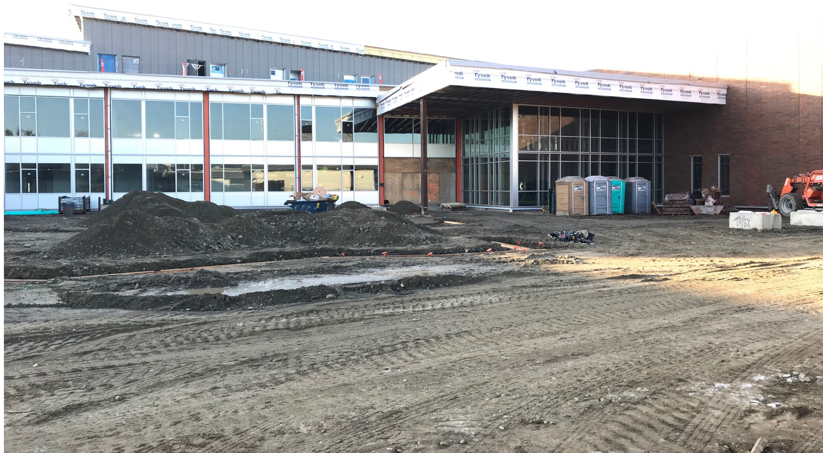
View of north elevation at student/PAC entry
