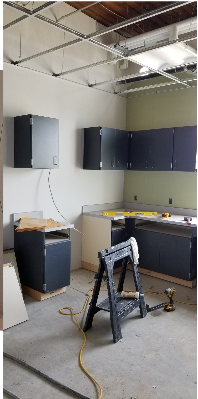
MTC Breakroom Casework
