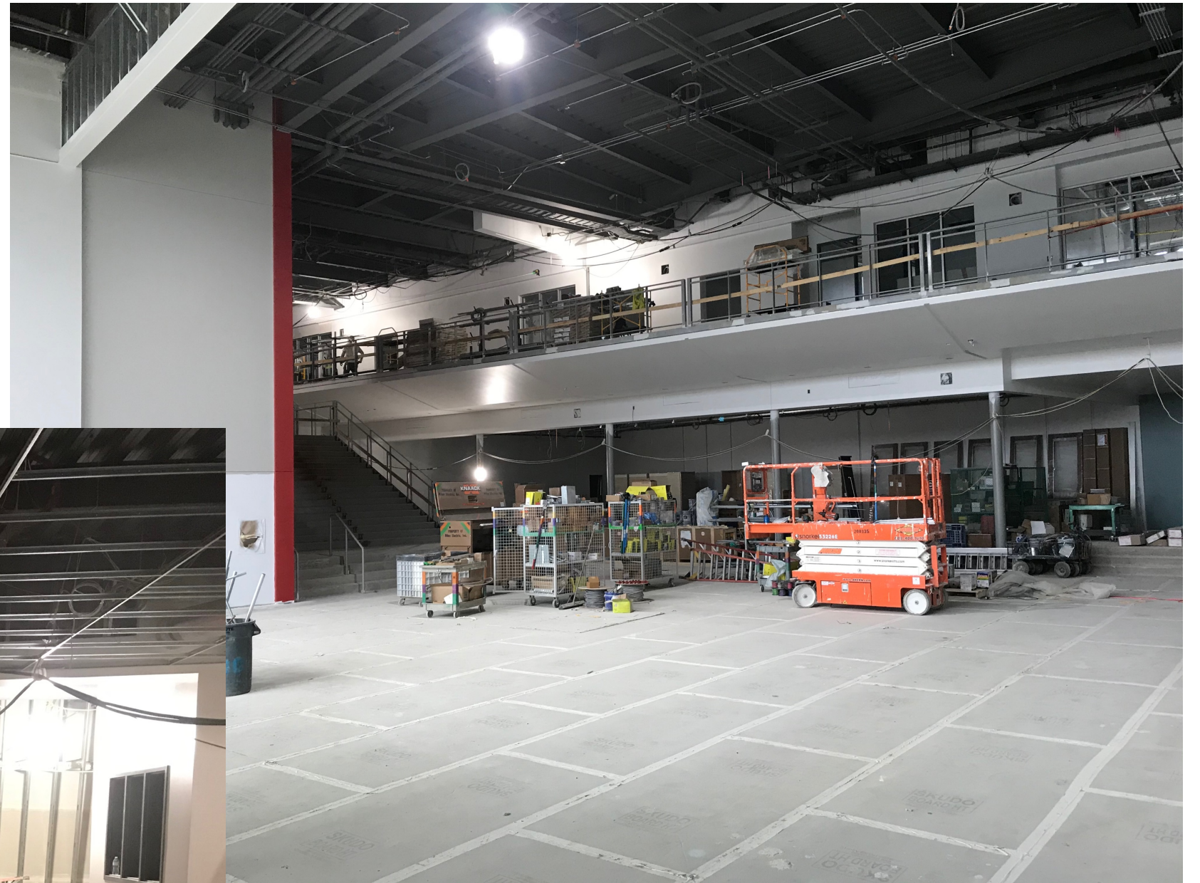
View from Commons to social stair and admin
