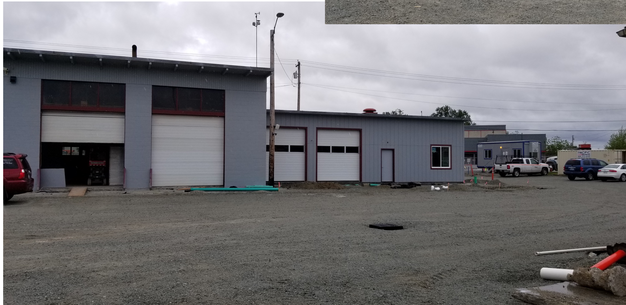
MTC Building View from the North
