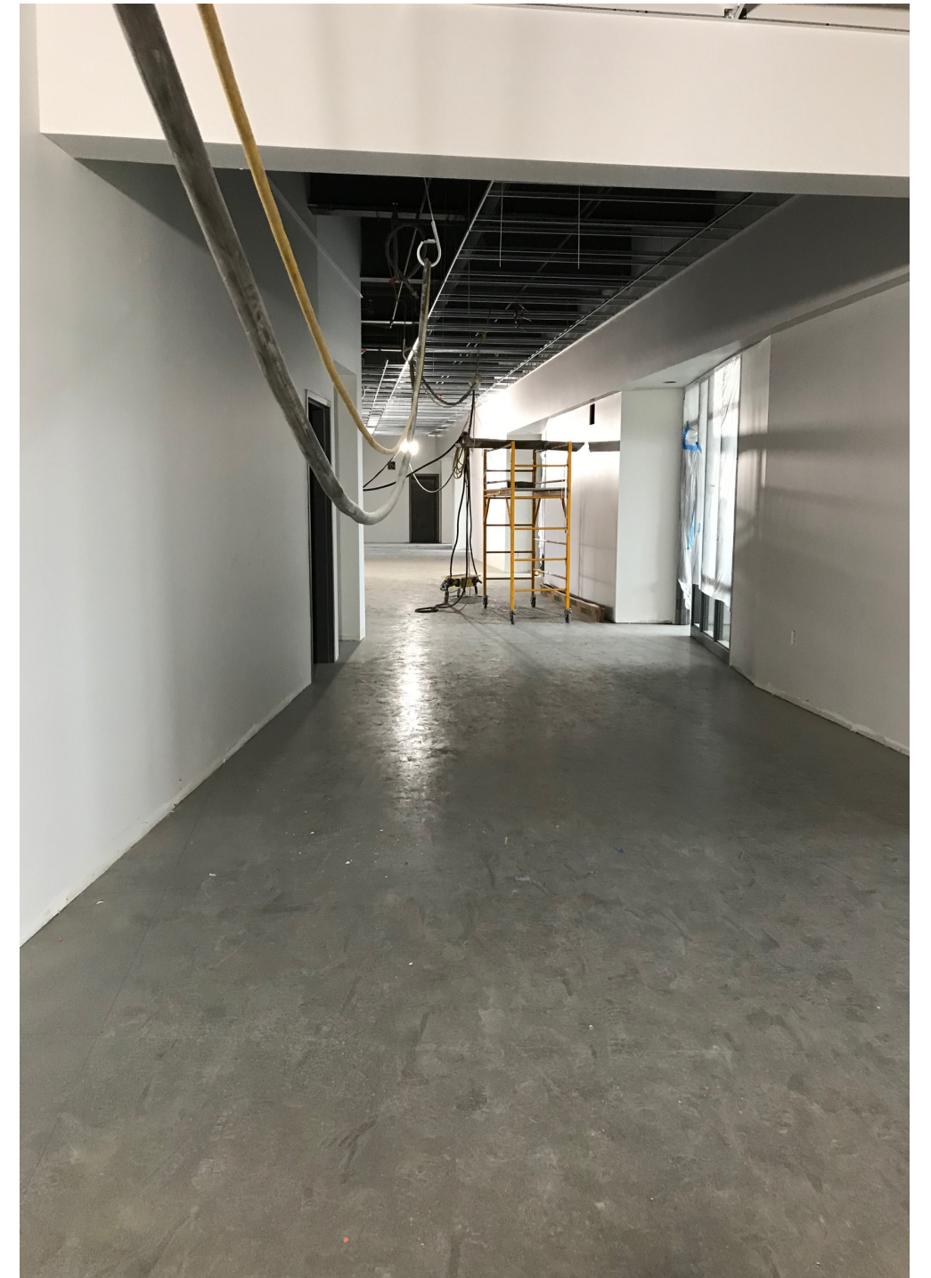
Classroom wing corridor
